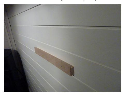
The ceiling absorber is easy to mount when the mounts are in place, just move it up in between the mounts and then slide it into position:
